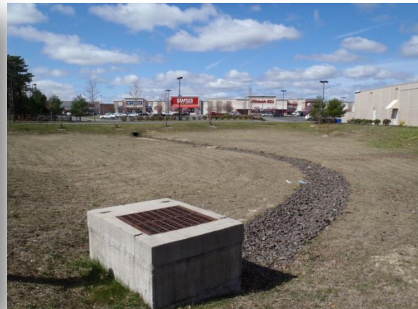
Gravel low flow channel
