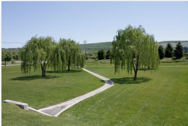
Concrete low flow channel
